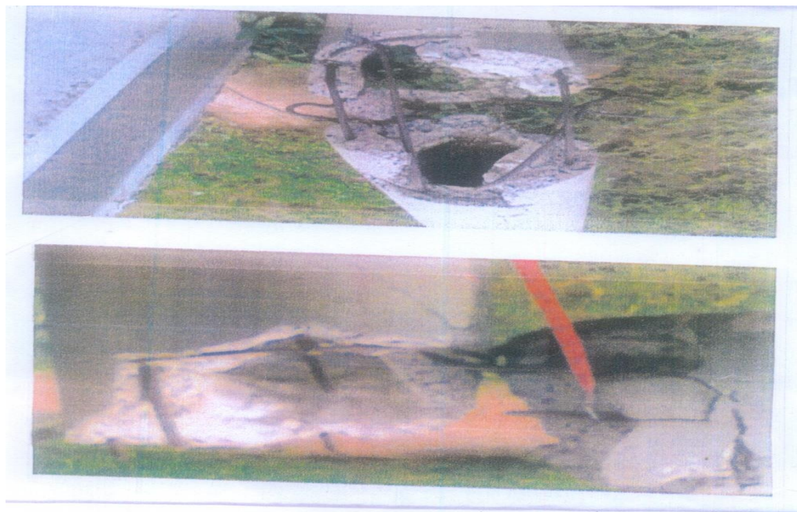
Plate II: Physical Crack on reinforced concrete pole, in Girei L.G.A, Yola.
