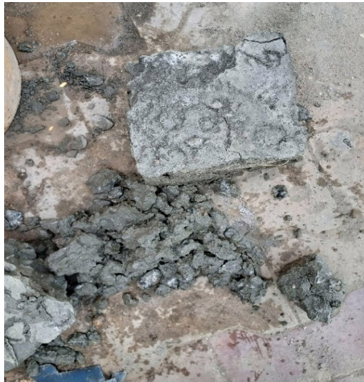
Plate 1. Disintegrated concrete cubes with NGP content of 1 and 1.2% during curing
